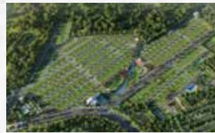
GREEN GROVES Nelamangala, Bengaluru
