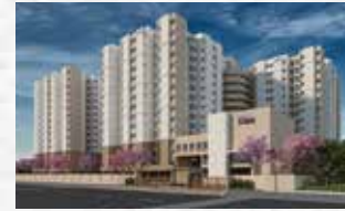
ASHRAYA Bengaluru-Mysuru Expressway Bidadi
